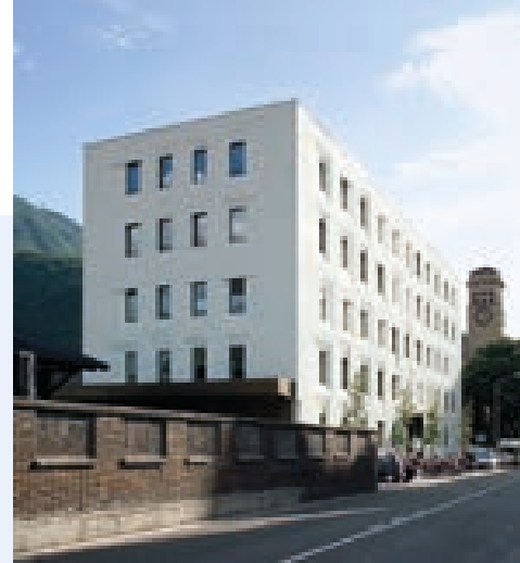
Silatex® Reflect application on exterior walls
